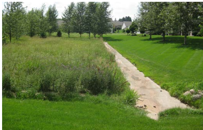
Figure 5: Concrete Drainage Channel
