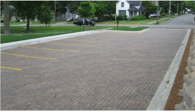
Figure 7: Permeable Paver Parking Lot
