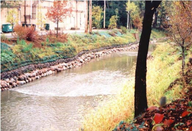
Figure 7: Stream Riffles/Slope Stabilization
