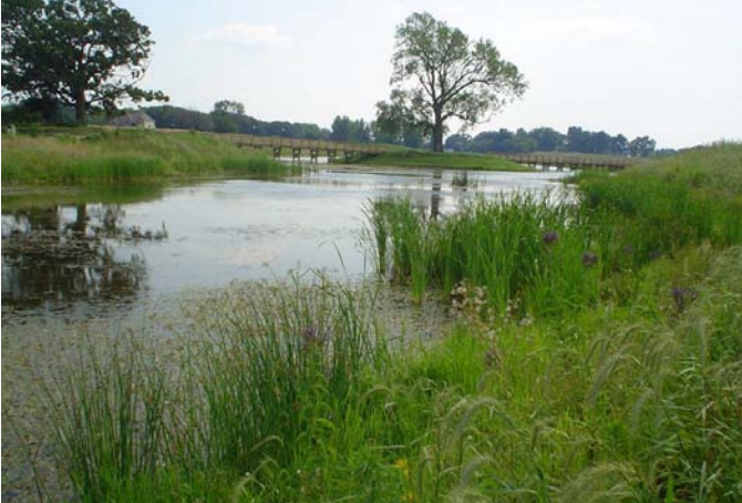
Figure 8: Naturalized Detention Basin
